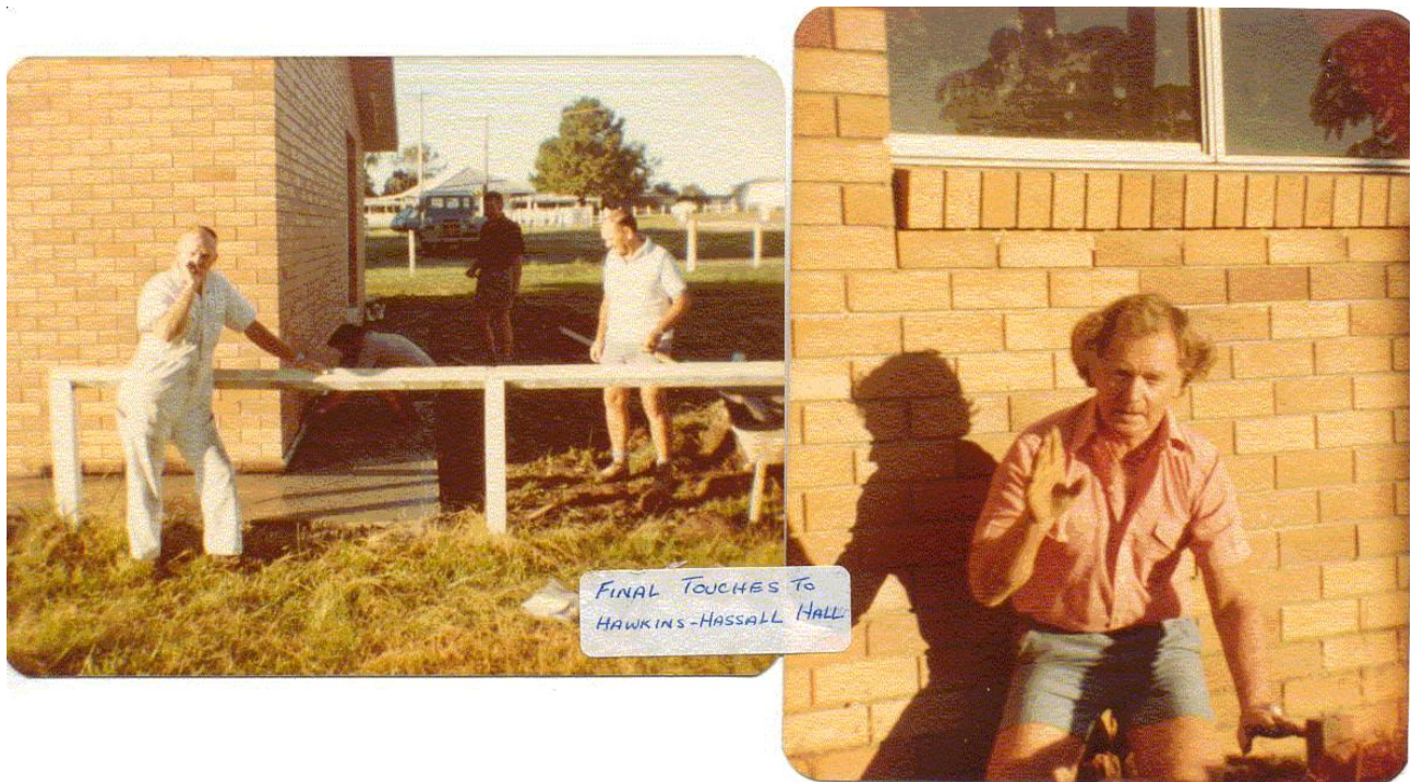
Completing the final touches for the Hawkins Hassall Hall.
