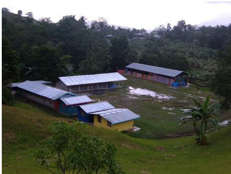
View of the children's accommodation, kitchen, and play area.
