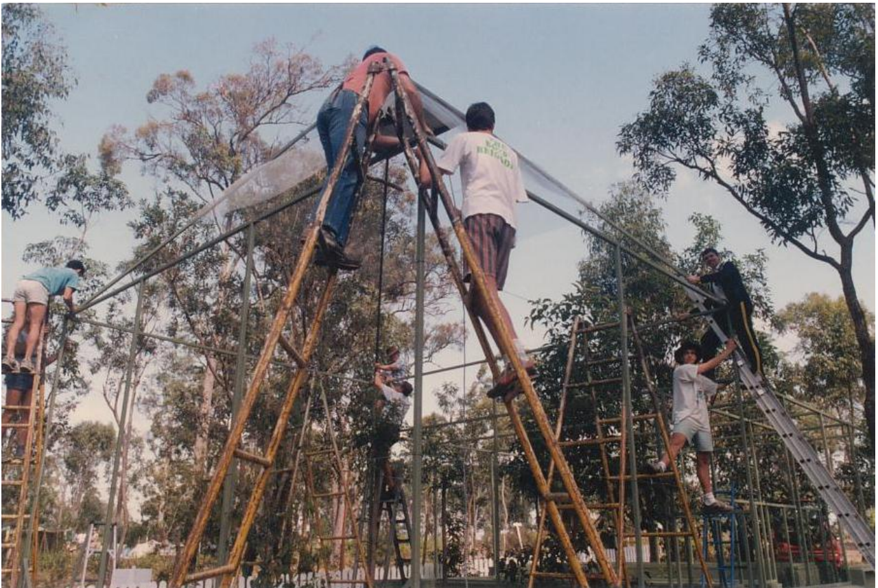
Work progresses and the roof goes on. It's a long way up there!
